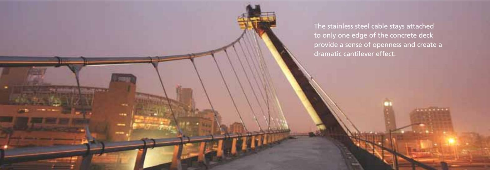
The stainless steel cable stays attached to only one edge of the concrete deck provide a sense of openness and create a dramatic cantilever effect.
