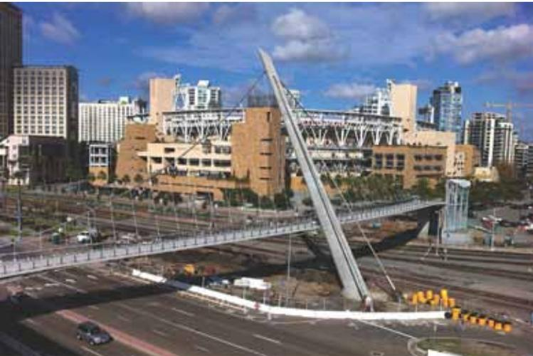
The Harbor Drive Pedestrian Bridge is a self-anchored suspension bridge with a 355-ft-long concrete main span situated in downtown San Diego adjacent to Petco Park, home of the San Diego Padres.
