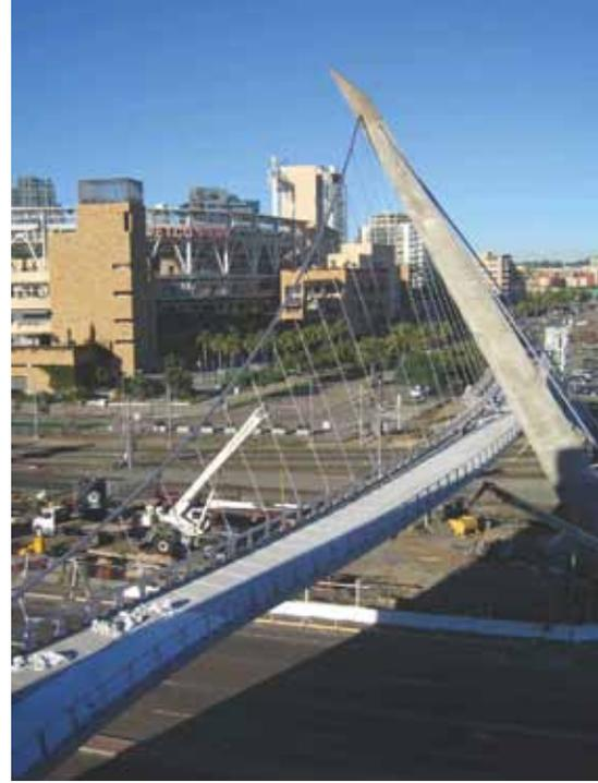
The 130-ft-tall concrete pylon is inclined at 30 degrees from vertical and reaches over the deck to produce a lateral curve in the main cable necessary to provide equilibrium to the structure.
