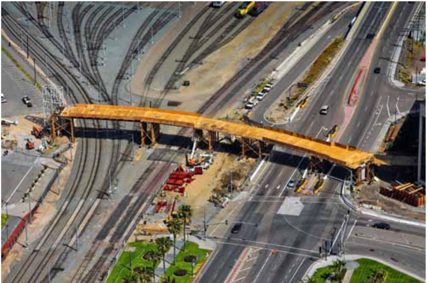
The concrete deck was cast in place on falsework that had to be designed to allow for over 3 in. of lateral displacement during stressing of the cables.
