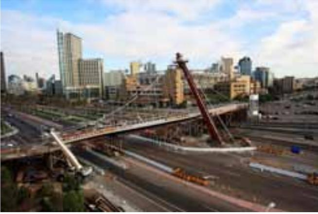
With both the deck and pylon built using in cast-in-place concrete, work on both proceeded simultaneously. Specially designed steel forms, shown in this photo, were used to construct the pylon in five lifts.
