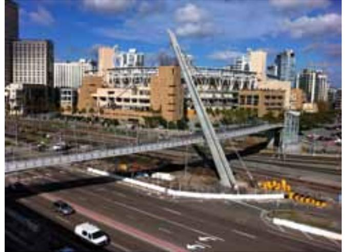
The Harbor Drive Pedestrian Bridge is a self-anchored suspension bridge with a 355-ft-long concrete main span situated in downtown San Diego adjacent to Petco Park, home of the San Diego Padres.
