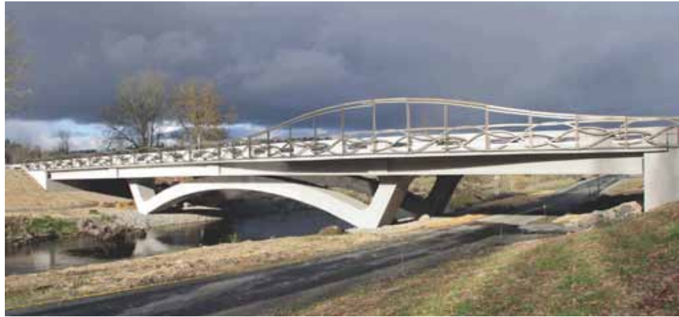
The York Bridge in King County, Wash., features a cast-in-place arch supporting a four-span precast concrete superstructure. The combination allowed the design to be consistent with other bridges in the area while maintaining the required structural integrity. Photos: King County DOT.
