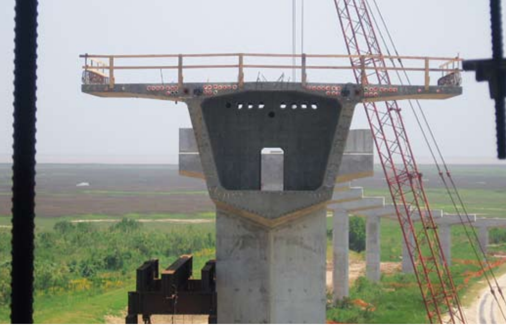
Cross section of the pier segment. Photo: Dean Van Landuyt, TxDOT.
