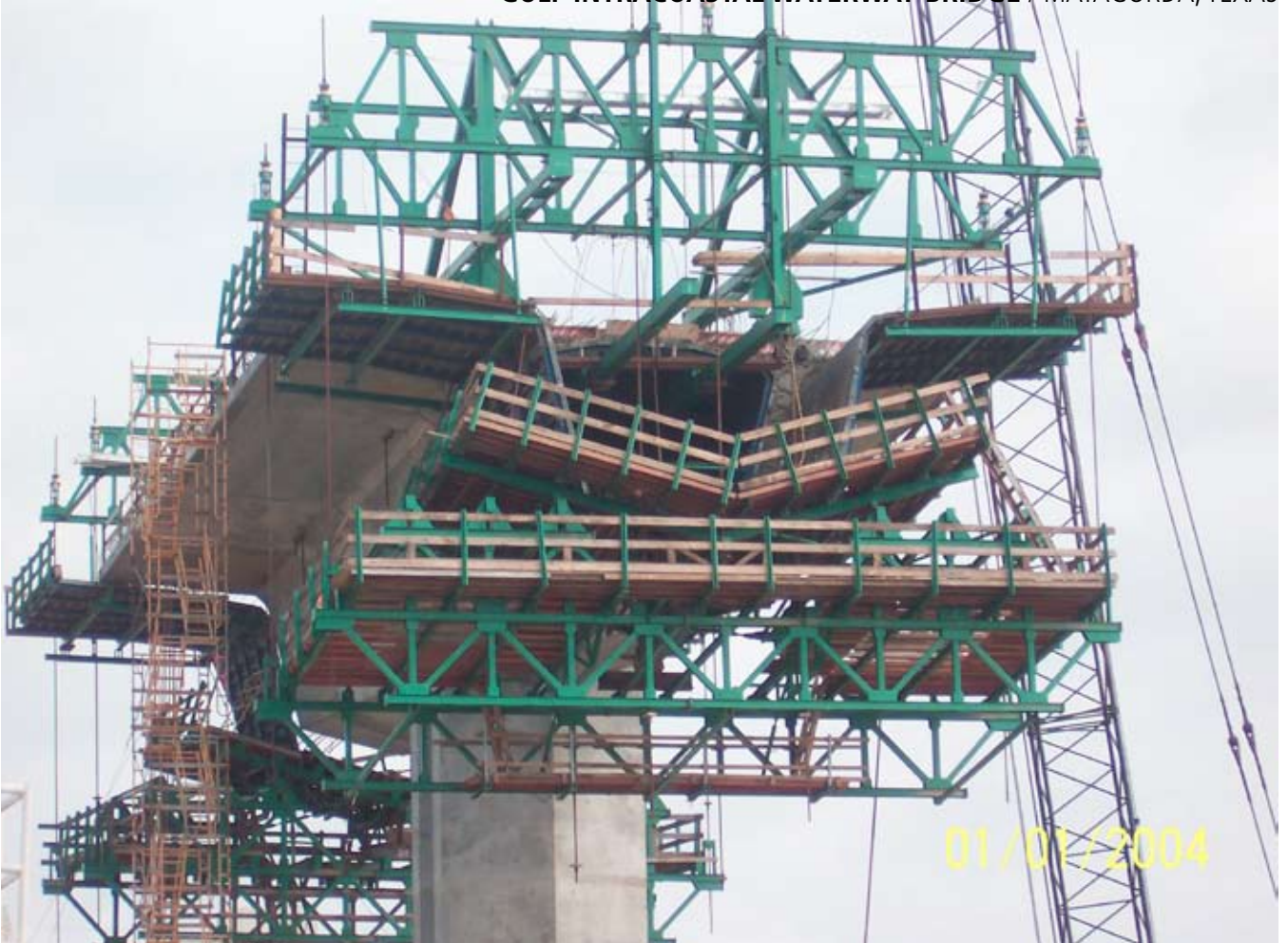
The traveler and formwork for the segmental unit. Photo: Michael Mann.
