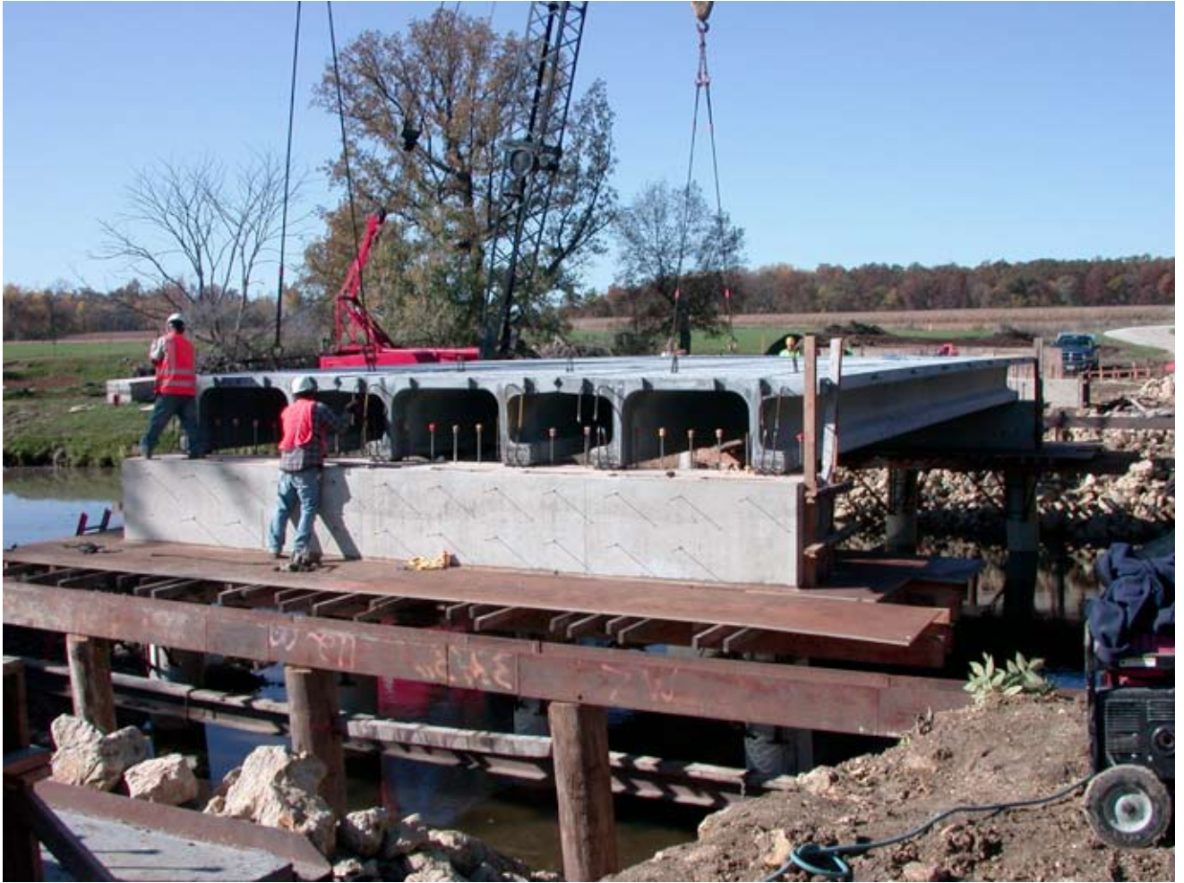
Three Pi girders were used to construct the bridge's center span.
