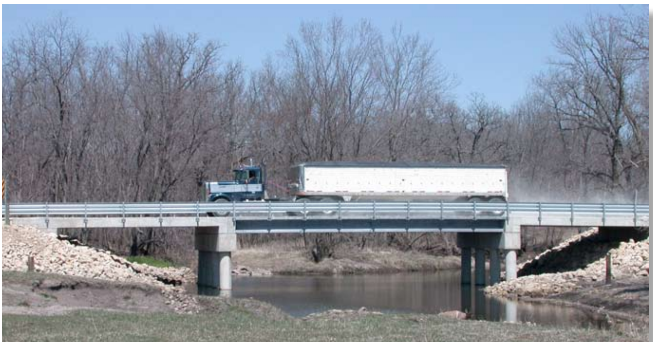
Three Pi girders were used to construct the bridge's center span.
