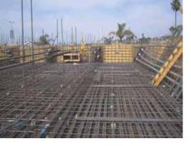
Each tendon contained thirty-seven, 0.6-in.-diameter strands. Concrete with a compressive strength of 4000 psi was used in the superstructure, columns, and piles. Other concrete used in the project had a compressive strength of 3600 psi.
