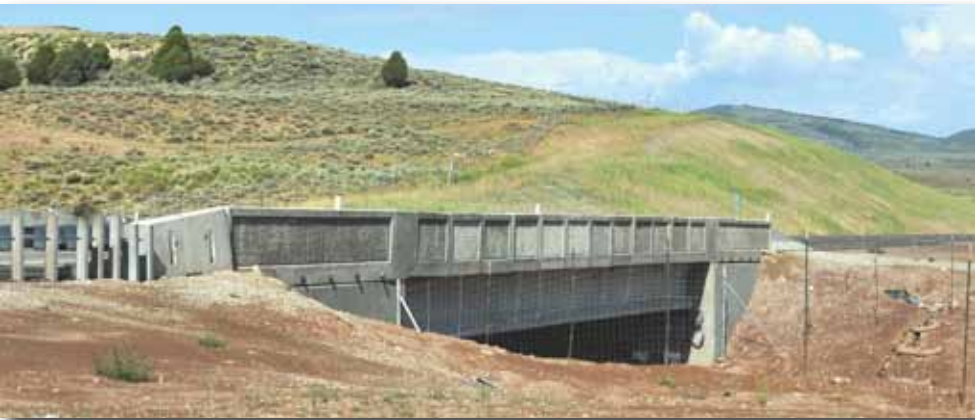
The Emma Park Bridge on U.S. 6 features precast, prestressed concrete girders and full-depth precast concrete deck panels. Photo: Utah Department of Transportation.
