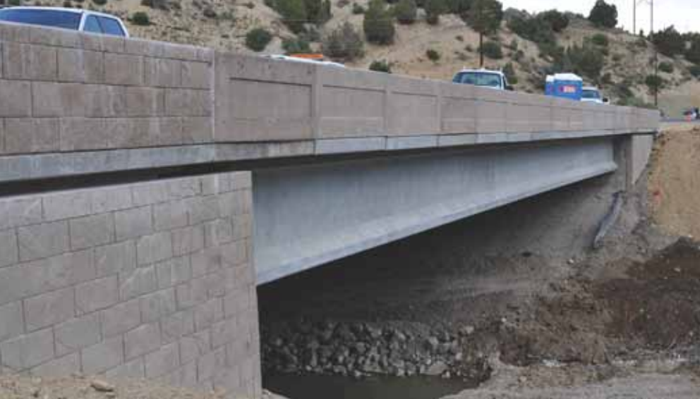
The Tucker Bridge on U.S. 6 is shown nearing completion. It is almost totally precast concrete. Formliner finishes were provided on the abutments, wing walls, and parapets. Photo: Utah Department of Transportation.
