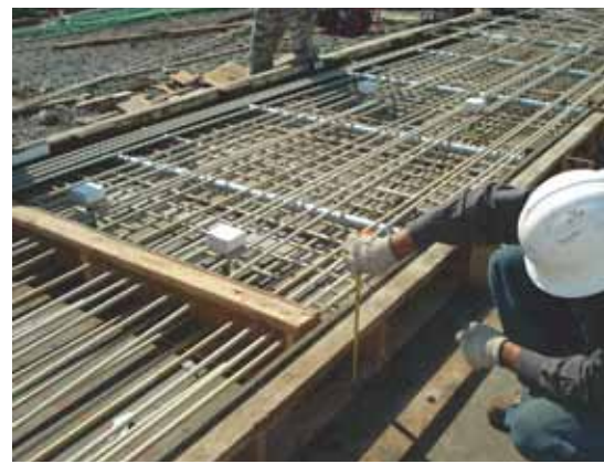
Shown during fabrication, deck panels are pretensioned in the plant. GFRP reinforcement is used in both top and bottom mats. Photo: Utah Department of Transportation.
