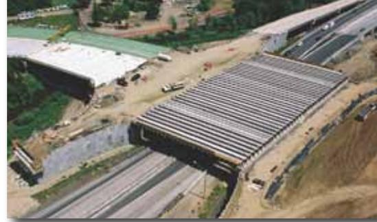
Looking toward the southeast shows the roadway structures approaching from the east and the bridge over Bear Creek. That bridge, the bridge over I-5, and the structures of the on and off ramps of northbound I-5 bear on abutments embedded in the MSE island constructed between the Interstate and the creek. The girders spanning over I-5 are not evenly spaced. Two groups of girders are more closely spaced to support the large pedestals and signal posts on the SPUI.
