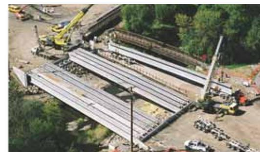
The longest span on the South Medford Interchange project was the 172-ft-long single span of the East Barnett Road Bridge over Bear Creek. It was one of two bridges on the project to use 90-in.-deep bulb-tee girders.
