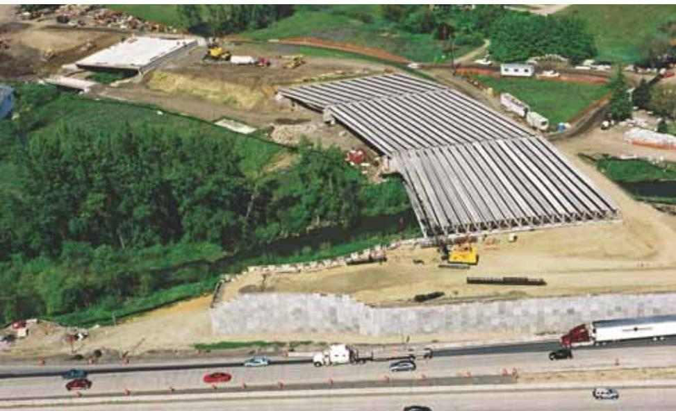
The three-span Highland Drive Bridge over Bear Creek is on a 700-ft-radius horizontal curve. Chorded spans with splayed girder lines accommodate the curve. Two additional bridges are shown in the background: the Highland Drive Bridge over Larson Creek and the Bike Path over Larson Creek.
