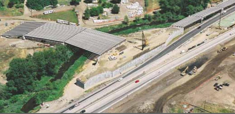
Another view of the Highland Drive Bridge over Bear Creek. The I-5 off ramp structure is at the upper right. H piles were driven through large concrete pipe sleeves embedded in the island fill for the abutments of the I-5 Bridge.
