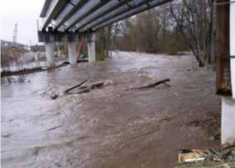
When Bear Creek flooded during construction, the concrete structures were unaffected resulting in no setbacks to the progress of the work. Photo: Wildish Construction Co.
