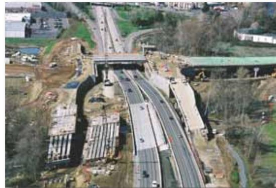
Looking to the north, Bear Creek crosses under I-5 at the location of the construction of the four bridges. The structure for the off ramp of northbound I-5 is nearly complete on the right. Northbound I-5 has been detoured to a temporary bridge. Southbound I-5 is using the finished northbound bridge. Work is ongoing on the bridges for southbound I-5 and the southbound on ramp. A portion of the original Barnett Road interchange can be seen at the top edge of the photo.
