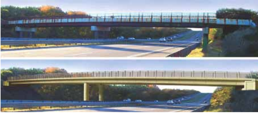
The new precast concrete channel bridge (bottom rendering) and the original steel I-girder bridge (top photo) and are shown for comparison. The new channel bridge provides more than 2 ft of additional clearance. Illustration: IBT.
