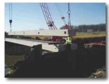
The erection of an adjacent precast, prestressed concrete box beam bridge on steel sheet pile abutments. This is a demonstration bridge in Blue Earth County, Minn.
