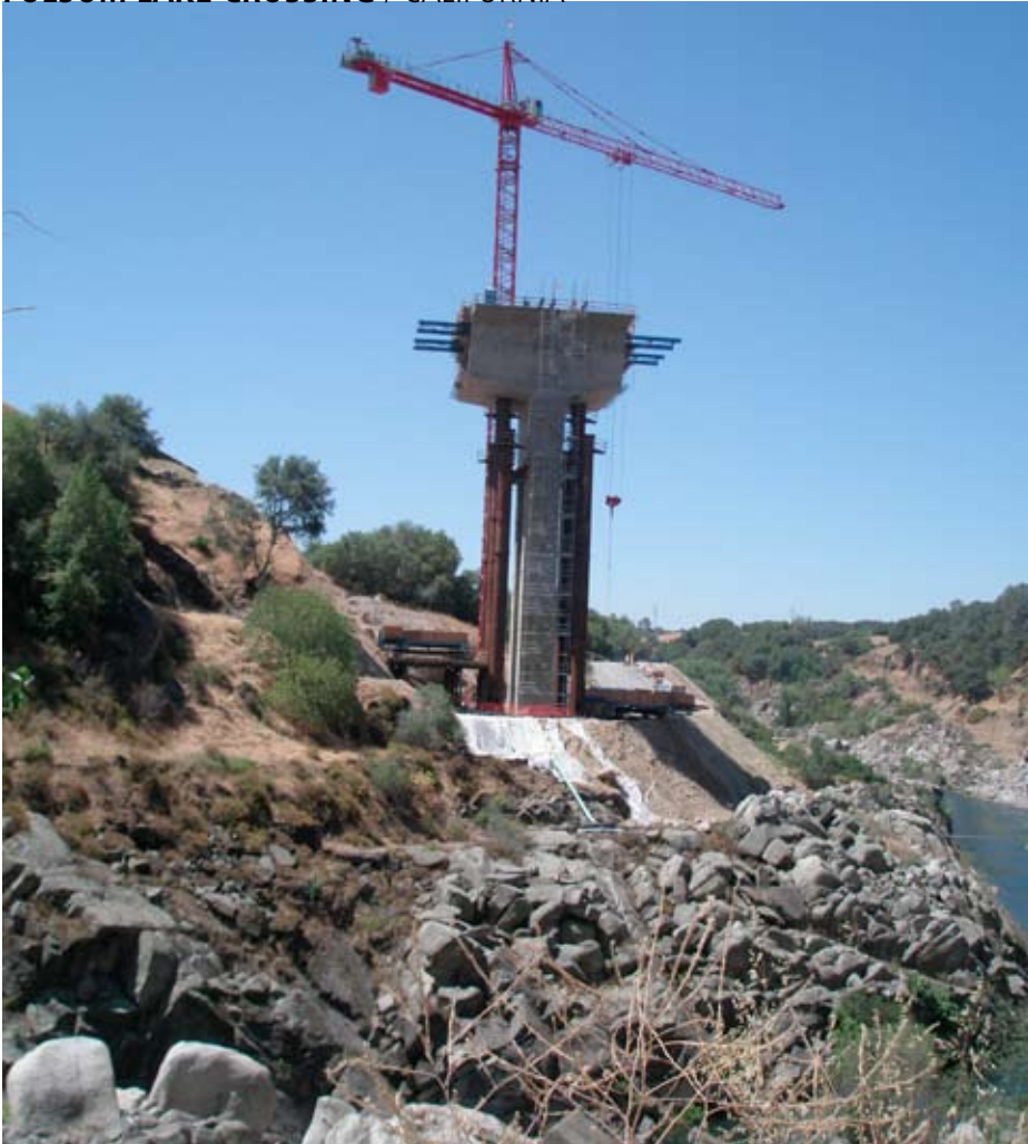
Pier 3 in June 2008.
