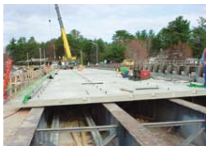
NHDOT's first use of precast, prestressed full-depth deck panels on the redecking of the Mosquito Bridge over Lake Winnisquam.
