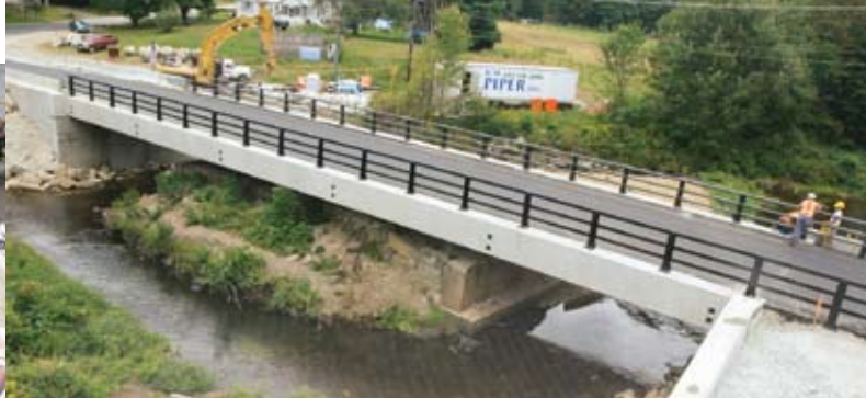
Eight days after the first precast footing piece was placed, the Mill Street Bridge in Epping was paved and opened to traffic.
