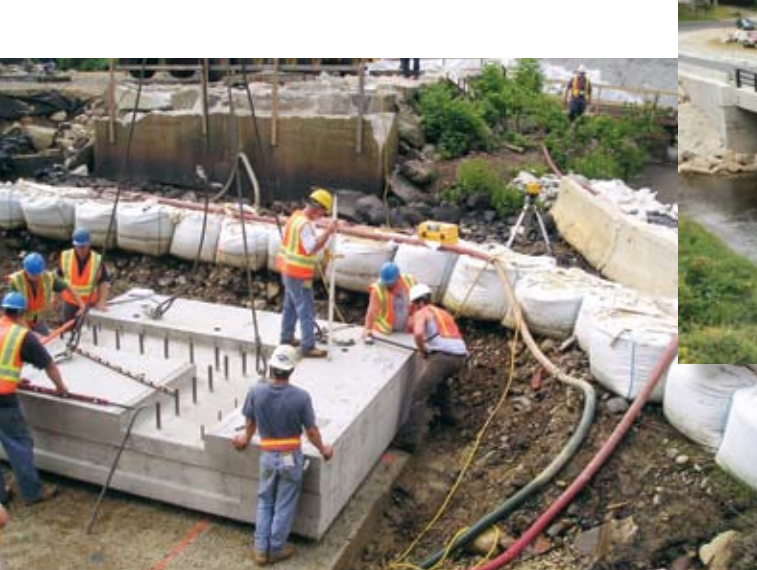
Placement of the first precast footing segment in NHDOT's first entirely precast bridge in Epping.
