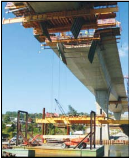
Concrete segmental cantilevers meet to form one of the 380' spans
