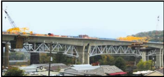
Span 2 at 380' (left) is within 4' of closure. 5 segments remain to complete Span 3, also at 380' (right)
