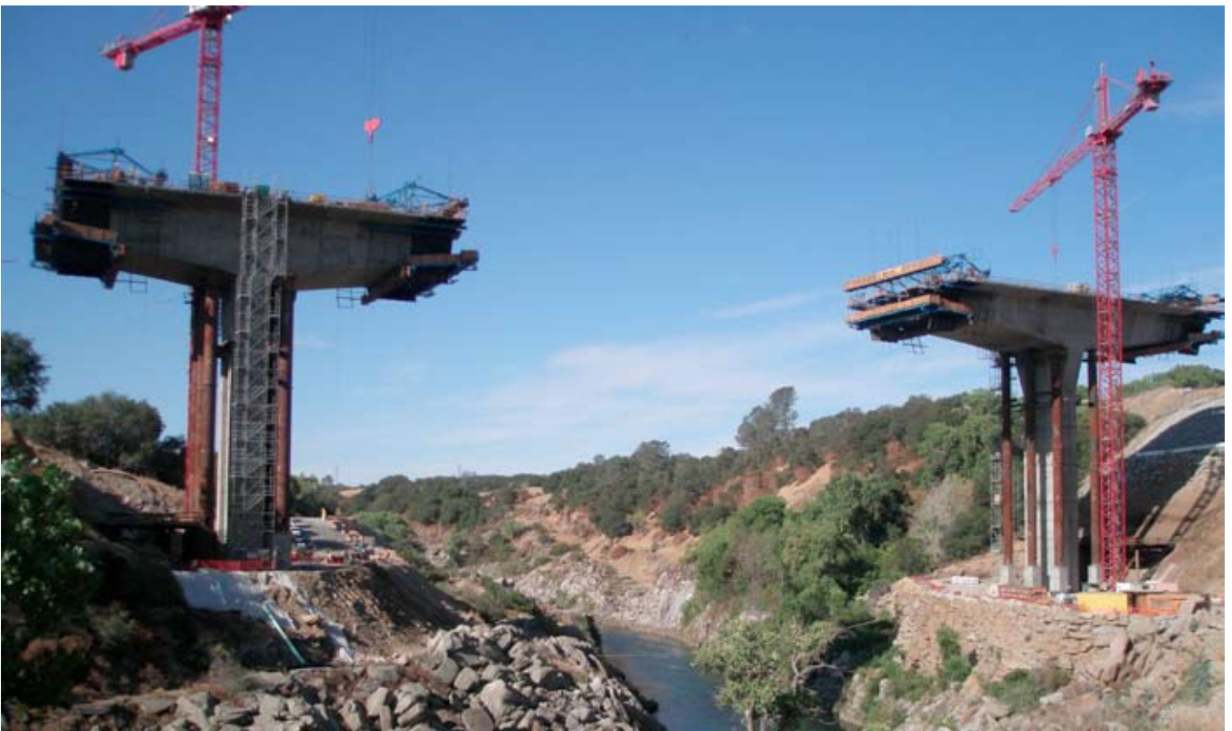
The cantilevers starting in August 2008.
