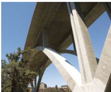
At the bents, each column pair appears as one column architecturally but operates as two columns functionally, with one of the pairs located on each side of the transverse deck joint. All photos: OBEC Consulting Engineers.
