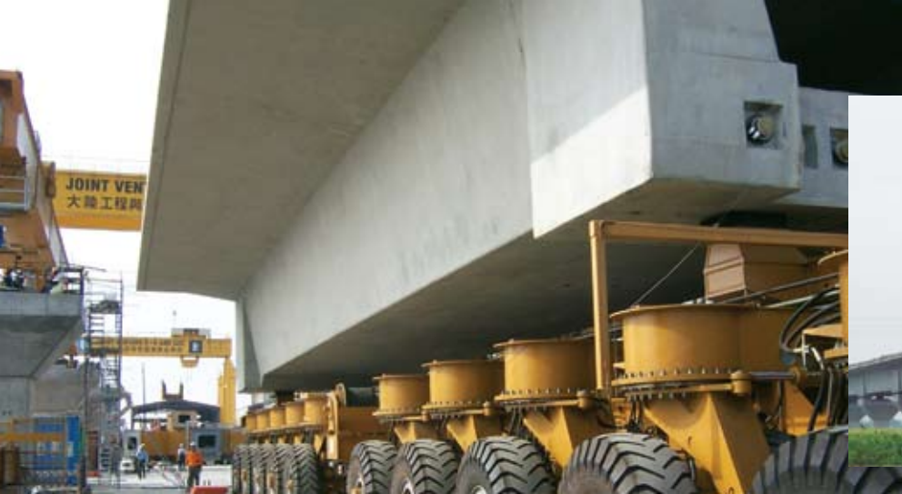
The superstructure of the Taiwan High Speed Rail comprises precast, post-tensioned concrete box girders, 3.25 m (10.7 ft) deep and up to 35 m (115 ft) long, weighing up to 780 tons.
