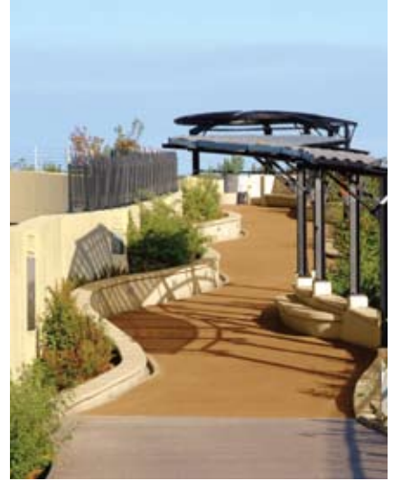
Boardwalks made with recycled plastic lumber span wetlands alongside the approach pathway. Overhead steel trellises lend a more personal scale. Photo: Natural Pave Photos.
