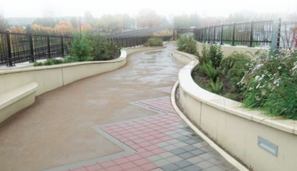
Meandering pathway leading away from the bridge. The walking surface is decomposed granite with a clear aggregate binder. Colored pavers were laid in symbolic Native American patterns. Photo: KPFF Consulting Engineers.
