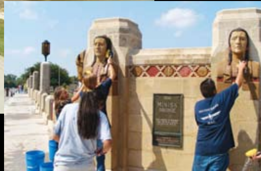
Community residents helping to restore some of the decorative sculptures on the Minisa Bridge.
