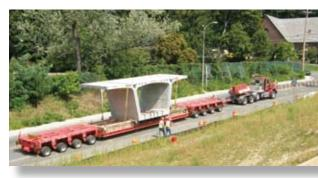
To protect the waterway near the site, precast concrete segments were barged from the precaster's plant in Cape Charles, Va., to a location several miles from the project and then hauled by specialized trailers to the site. Photo: Will Brown.
