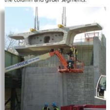
Ironworkers align the couplers for the post tensioning bars as they set the precast concrete column cap segment at pier 7. Photo: Renata Magoc.
