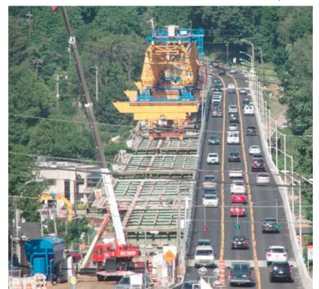
After the north side of the bridge was constructed, the gantry crane was shifted to the south to remove the steel frame of the existing bridge. Photo: Rich Lorenzen.
