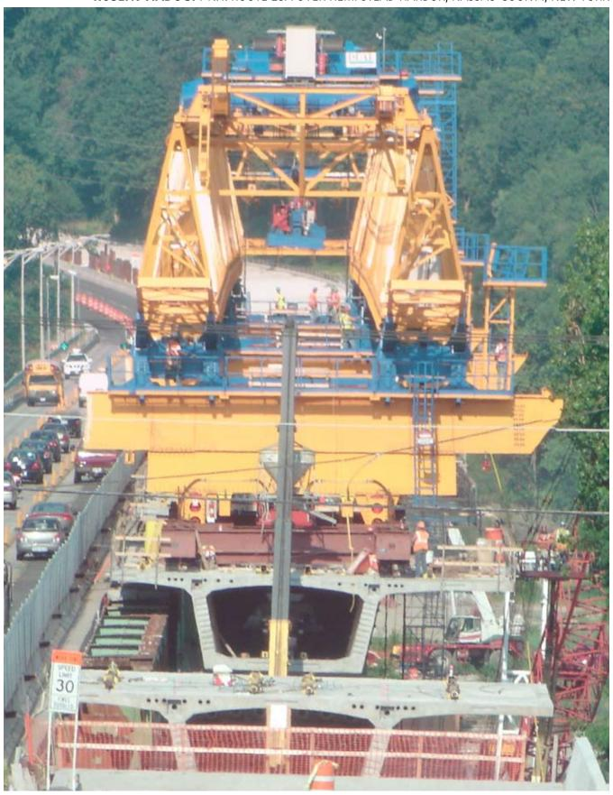
Concrete is placed at the closure pour at pier 7 using a crane and bucket while the gantry is positioned at piers 6 and 7. In the foreground are the pier 8 pier table and the east abutment. Photo: Rich Lorenzen.
