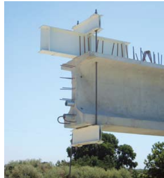
Strongbacks were used to support the drop-in segments. Photo: Port of Stockton.
