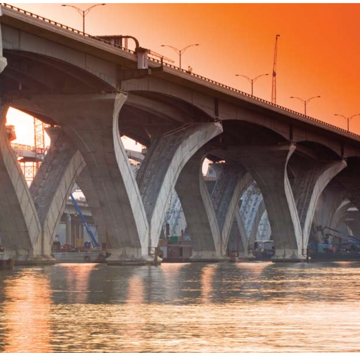
To blend the new Woodrow Wilson Memorial Bridge with other Potomac River crossings, Parsons' designers used V-shaped precast concrete piers with curved legs. Photos: Parsons.
