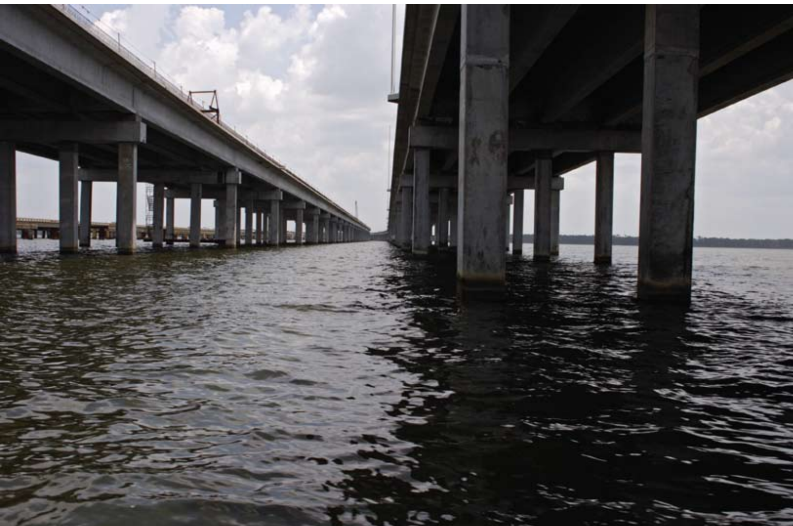
Low-level pile bents.
