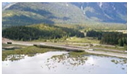
Washington—I-90 Snoqualmie Pass East Project, stream crossing. Photo: WSDOT.
