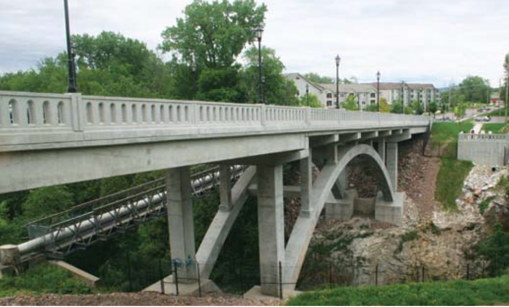
The 300-ft-long bridge features precast, prestressed concrete box beams and slabs with cast-in-place concrete arches, piers, floor beams, and deck. The arch supports six intermediate 22-ft-long spans that used 1-ft-deep precast concrete solid slabs.
