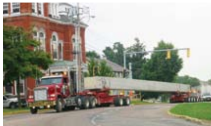
Remote-controlled, steerable dollies were used to maneuver the 104-ft-long precast concrete box beams. Photo: J.P. Carrara & Sons
