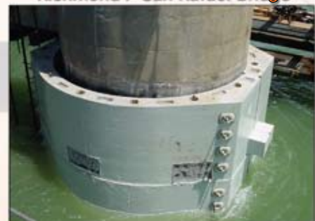
Richmond / San Rafael Bridge
