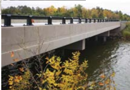
TH 72 over Tamarac River. (Three-span precast, prestressed inverted "tee" beam deck)
