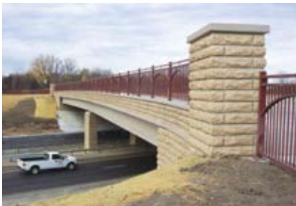
Pioneer Trail over TH 169, West Bloomington/Eden Prairie. (Two-span prestressed concrete girder bridge)
