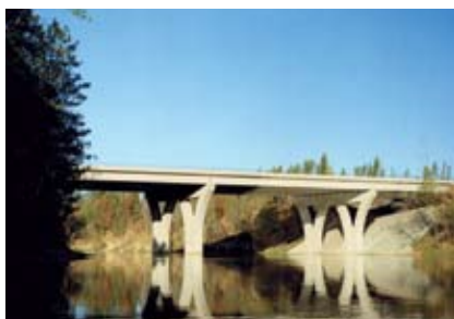
TH 371 over the Mississippi River, near Brainerd. (Three-span prestressed concrete girder bridge)
