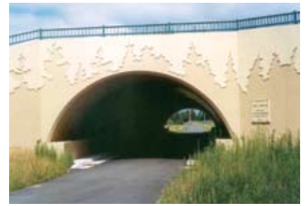
TH 210 over Paul Bunyan Trail, Brainerd. (Precast concrete arch)
