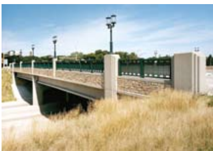
36th Avenue North over TH 100, Robbinsdale. (Two-span prestressed Concrete girder bridge)
