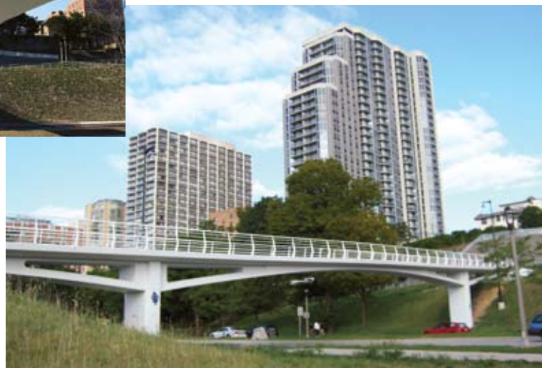
A berm was created up to the edge of the bridge along the end facing the lake to avoid the need for a long stairway and to lower budget needs.
