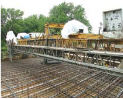
Reinforcing steel and cable ducts just before the concrete placement.
