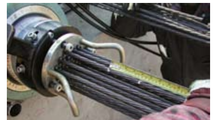
After the concrete has gained strength, the cables are post-tensioned and strand elongation measured.
