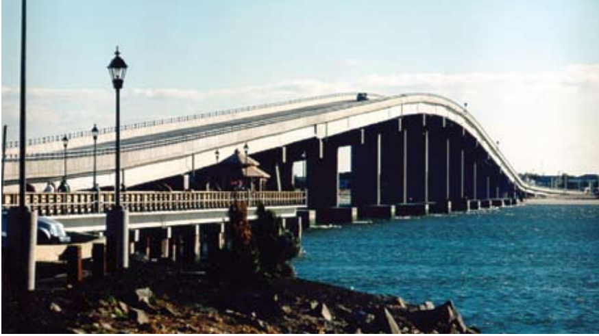
The Ocean City-Longport Bridge, N.J., included three-span continuous units made from modified AASHTO Type VI 90-in.-deep spliced post-tensioned girders with a maximum span length of 222 ft. Photo: ©PB.
