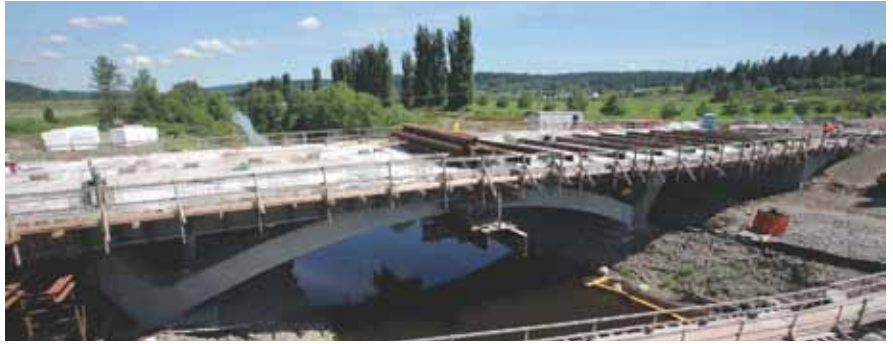
The cast-in-place deck features epoxy-coated reinforcing bar to provide corrosion protection.
