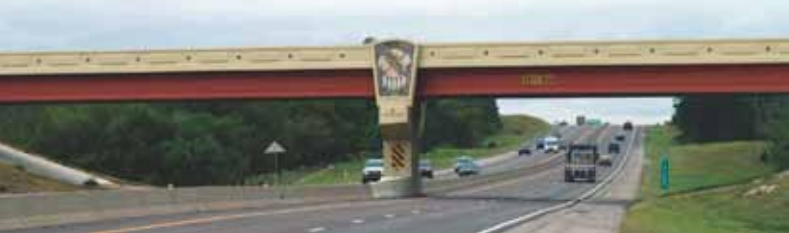
The two-span, precast, prestressed concrete SH 102 Bridge over Turner Turnpike near Wellston was the state's first structure to feature a special aesthetic treatment consisting of colored components and an embedded concrete theme cap at the juncture of the center pier and superstructure.
