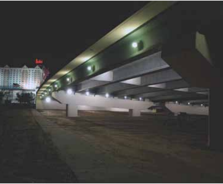
At the Biloxi Bay Bridge in Mississippi, a pedestrian pathway and small park engage the shoreline and allow for beachcombers to pass under the structure.
