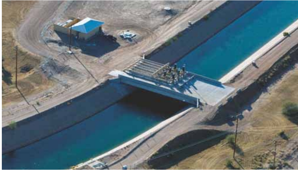
Aerial view of the bridge-mounted pumping station. All photos: Central Arizona Project/Central Arizona Water Conservation District.
