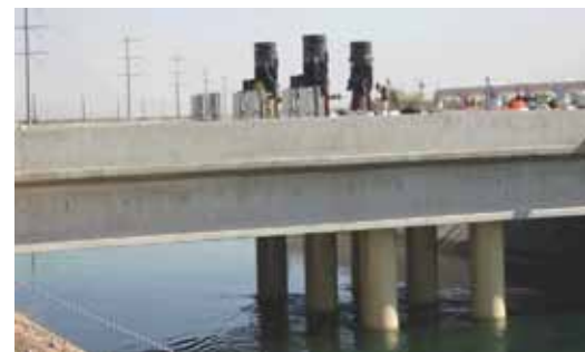
All six pump cans extend below deck into the canal and three pump-motor assemblies are mounted above.
