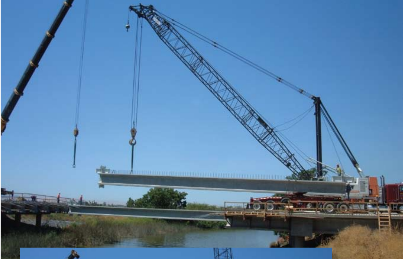
Cranes on the pier segments were used to erect the drop-in segments. Photos: Port of Stockton
