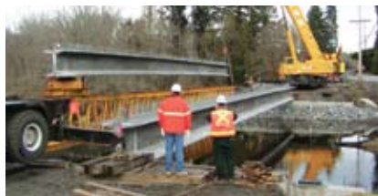
Old Highway Bridge No. O-9, originally built in 1923, was replaced in 2007 with a 110-ft-long, 42-ft-wide precast, prestressed concrete bridge.
