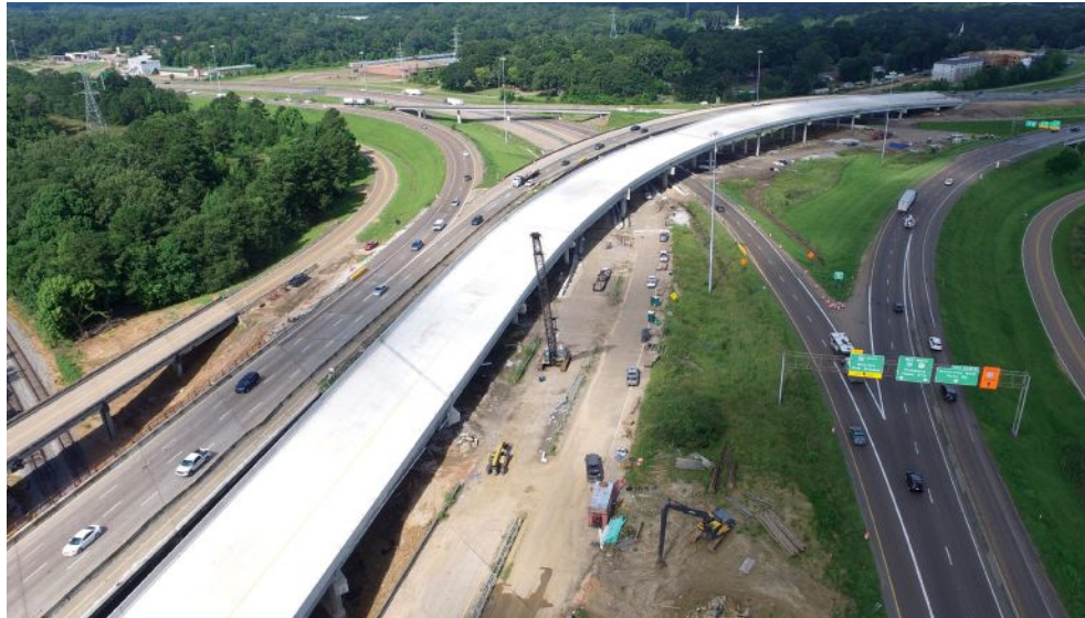
Aerial view of completed bridge before opening to traffic, looking west. Photo: Mississippi Department of Transportation.
