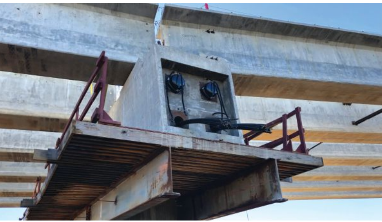
Bent 8 has a 65-ft-long straddle cap beam that required two stages of post-tensioning. The first stage was for the self-weight of the cap beam (already completed); in the second stage, tendons were tensioned shortly after the girders were set (not yet completed). Photo: HNTB Corporation.
