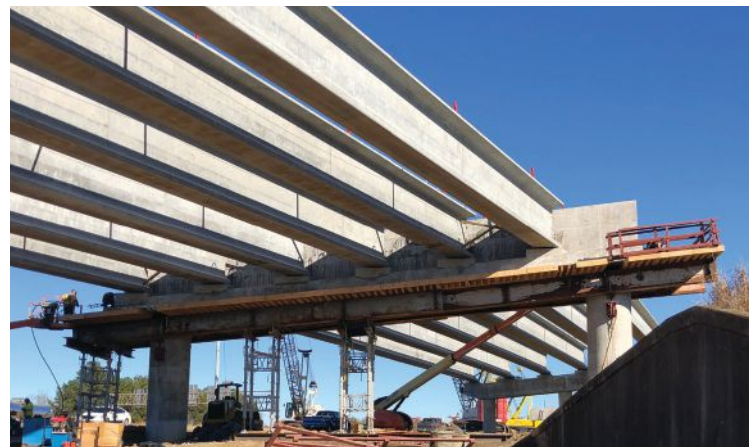
Prestressed concrete girders sit on the inverted-tee straddle cap beam at bent 9 before placement of the full-depth continuity diaphragm. Each of the two straddle cap beams has four tendons with thirty-seven 0.6-in.-diameter strands that were tensioned from only one end. Photo: HNTB Corporation.
