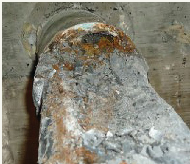
Figure 3. Corrosion of an external post-tensioned tendon at a location of soft, moist grout. Photo: Structural Technologies.
