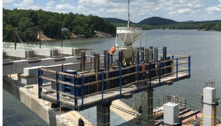
Cast-in-place concrete cap construction.
