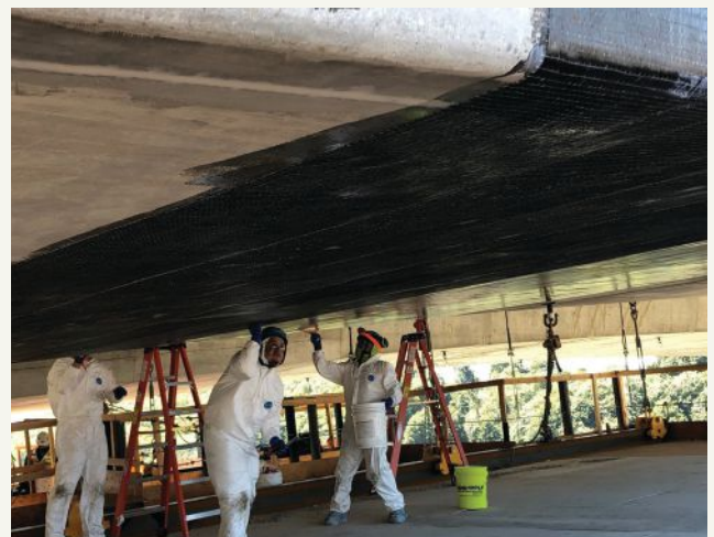
Figure 6. Carbon-fiber-reinforced polymer (CFRP) being installed to strengthen a concrete segmental bridge. Proper design, detailing, and installation is required for a CFRP strengthening system. Photo: Structural Technologies.
