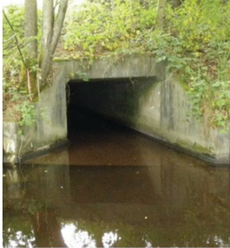
Figure 4. Church Creek, tributary to the Stillaguamish River. The old crossing (left) was replaced with a larger structure (right) to reduce channel velocities and increase depth for migrating salmon.
