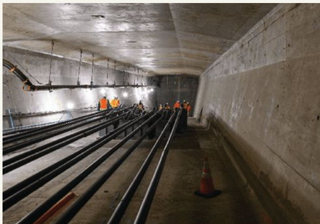
Figure 7. External post-tensioning tendons being installed to strengthen an existing concrete segmental bridge. Photo: Seattle Department of Transportation.
