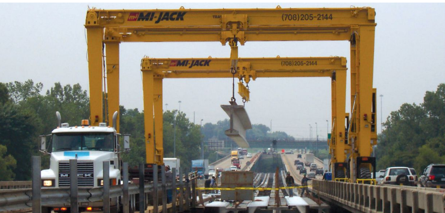
Figure 1. With the ability to straddle the gap between the existing structures, a rubber-tired gantry crane allowed work to progress on the Interstate 65 bridge over the Alabama River without lane closures. It also eliminated the need to transport cranes to other areas of the project. All Photos: Mi-Jack Products.
