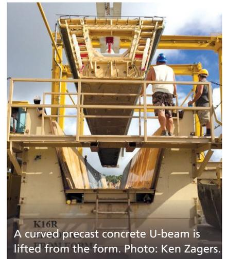
A curved precast concrete U-beam is lifted from the form. Photo: Ken Zagers.
