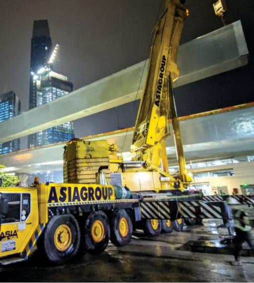
A 230-ft-long ultra-high-performance-concrete (UHPC) U-girder being erected for the Setiawangsa-Pantai Expressway, part of the Duta-Ulu Kelang Expressway system in Kuala Lumpur, Malaysia. UHPC is a relatively recent innovation in the precast concrete industry. Photo: Dura Technology.
