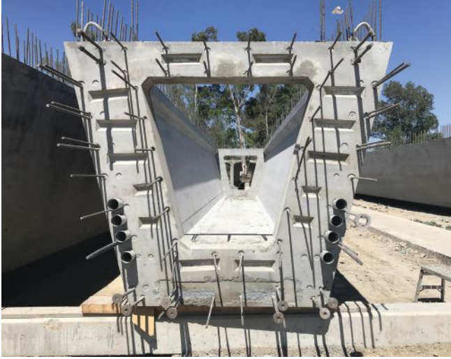
Typical precast concrete straight U-girder segment. Photo: WSP.
