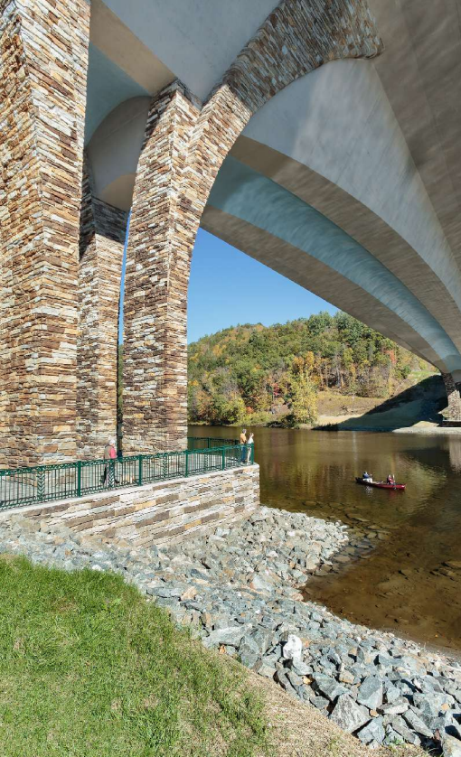
The Interstate 91 Brattleboro Bridge in Brattleboro, Vt., received a 2018 Concrete Reinforcing Steel Institute HONORS Design and Construction Award. The 1036-ft-long, three-span segmental, cast-in-place concrete box-girder structure features a 515-ft-long main span that was designed for a 150-year service life. Photo: © Adam Cohen 2017, Figg Engineering Group.
