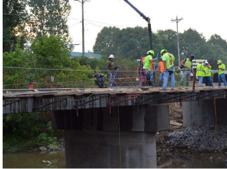
A construction crew in Franklin County, Ky., places concrete for the deck of a new concrete bridge that is part of the Bridging Kentucky program.
