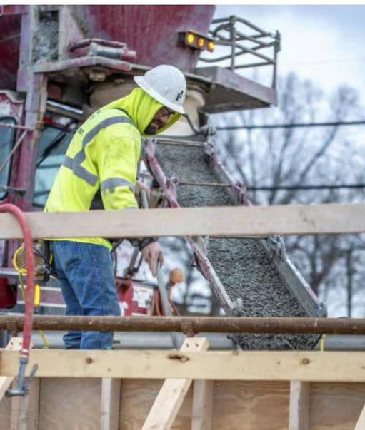
A construction worker assists in placement of a new concrete deck on a bridge in Nelson County, Ky.
