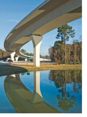
The North Interchange Project in Jacksonville, Fla., features a precast concrete segmental box-girder overpass. The concrete segmental design resolved challenges in design and construction created by difficulties with placing the overpass over existing roadways and limited right-of-way. It was the first project to specify duct couplers for joining internal post-tensioning ducts, which is now a standard technique.
