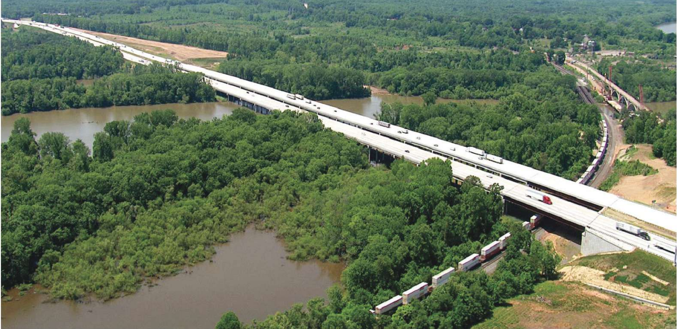
The I-85 Yadkin River Veterans Memorial Bridge near Salisbury, N.C., featured dual 2900-ft-long structures. Photo: Aerophoto.
