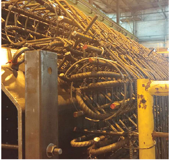
Detail of reinforcing steel cage for hollow concrete tower designed to resist blast loading.
