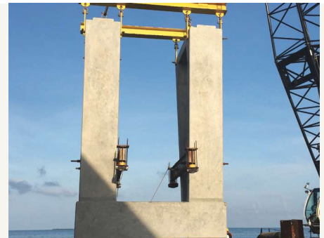
New V-pier being lifted and placed onto the temporary support system. Hydraulic jack and roller assembly is mounted on the column legs.
