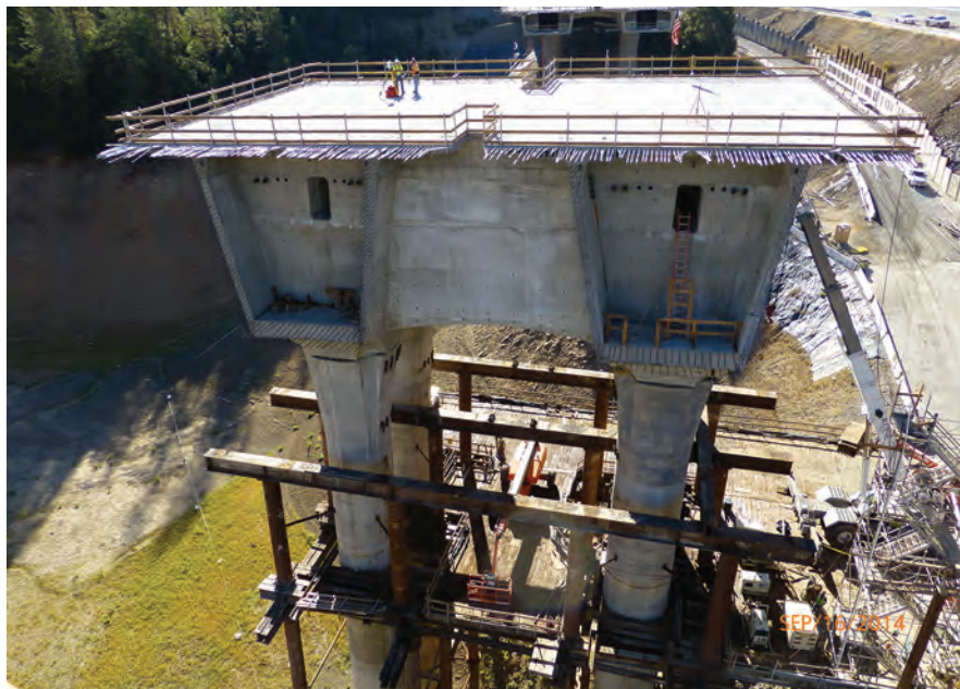
Massive columns are monolithic with the heavy pier cap.
