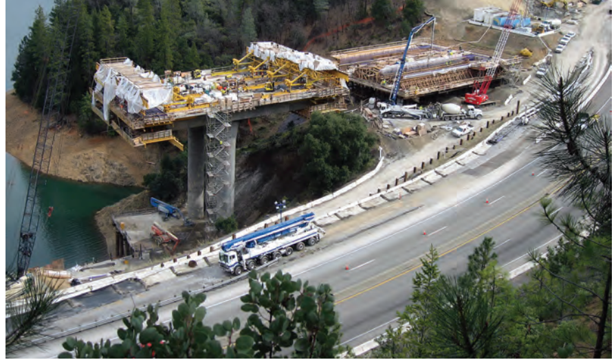
Falsework was used near the bridge abutments.
