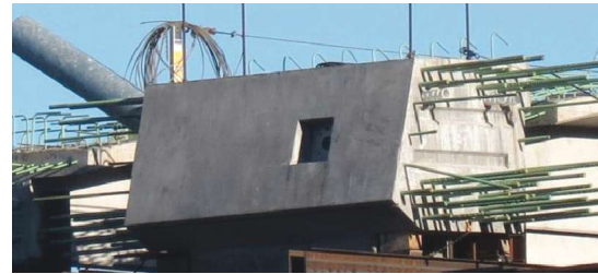
Design innovation – precast concrete anchor blocks. Photo: Brayman Construction Corporation.
