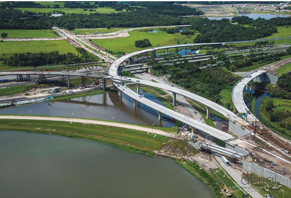
Aerial view of both Ramps H and I. Photo: SEMA Construction.
