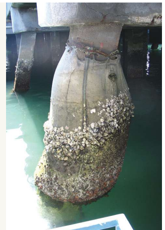
Figure 2. Fabric form jacket with concrete fill.
