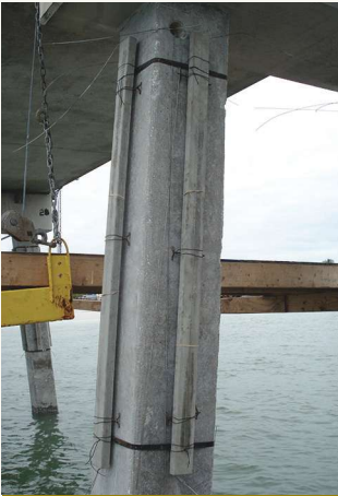
Figure 6. Dry jacket that includes alkali-activated anodes on the pile prior to jacketing (bulk zinc anode not shown).
