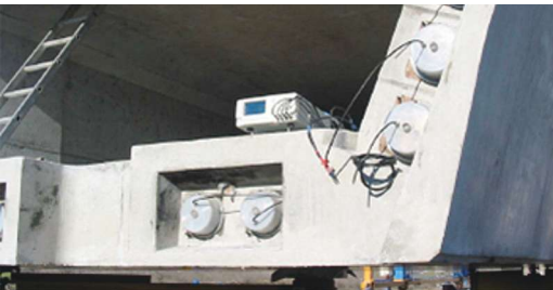
Figure 2. Monitoring at post-tensioning anchorage.
