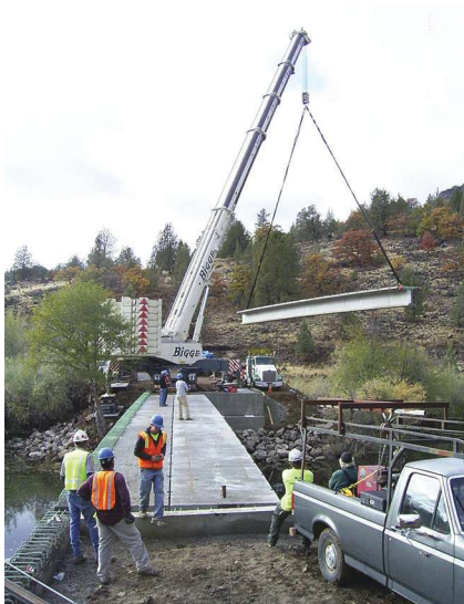
Decked bulb-tee being erected by a single pick. Photo: Morrison Structures Inc.
