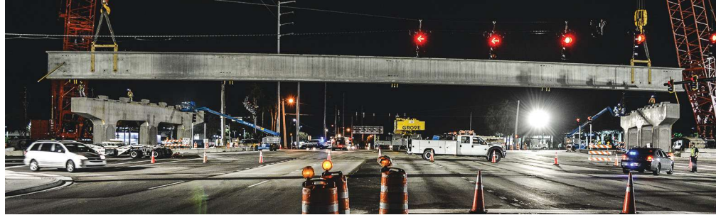
At 209 ft, the main-span beams are the longest single-piece precast, pretensioned concrete beams in the United States. Photo: The Lane Construction Corporation.
