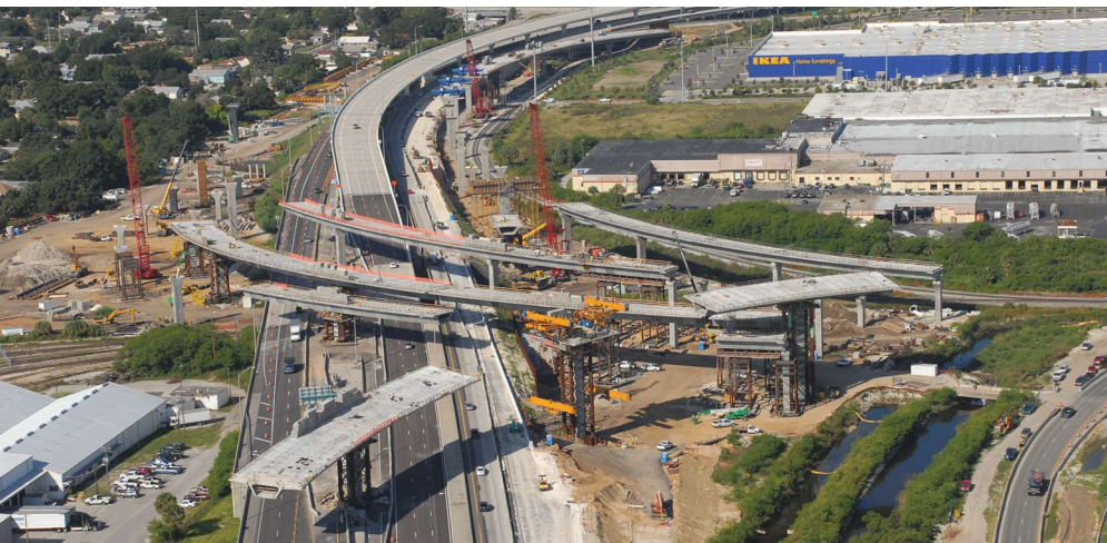
The 2765 precast concrete segments and 11 precast concrete bulb-tee girder bridges were used for the I-4 Lee Roy Selmon Expressway Connector project. Photo: PCL Civil Constructors and Archer Western Construction, joint venture.
