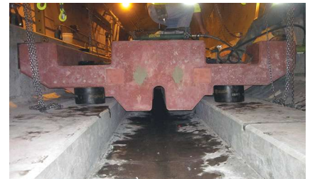
The University Link Extension features a 440-ft-long stretch of vibration-damping rails under Capitol Hill that "float," or rest, on 7.5-in.-thick elastomeric isolation bearing pads.
