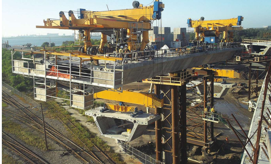
The precast concrete segments and precast concrete bulb-tee girder bridges of the I-4 Lee Roy Selmon Expressway Connector project use more than 500,000 ft 2 of concrete bridge decks. Photo: Walsh Group.
