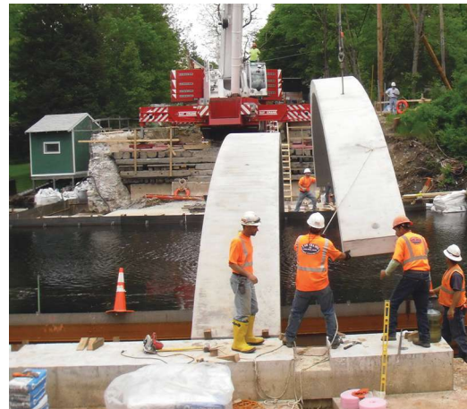
Installation of the precast concrete arches for the Willow Street Bridge. Photo: Matt Hopkinson.
