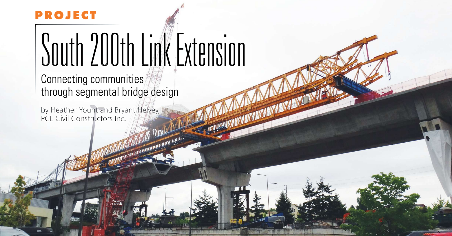
Installation of the last segments of the South 200th Link Extension. Photo: PCL Civil Constructors Inc.
