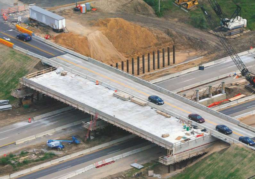
M-50 over I-96 traffic on new superstructure in temporary alignment. Photo: Michigan Department of Transportation.
