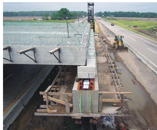
Temporary pier and span 1 beams in sliding track. Photo: Michigan Department of Transportation.
