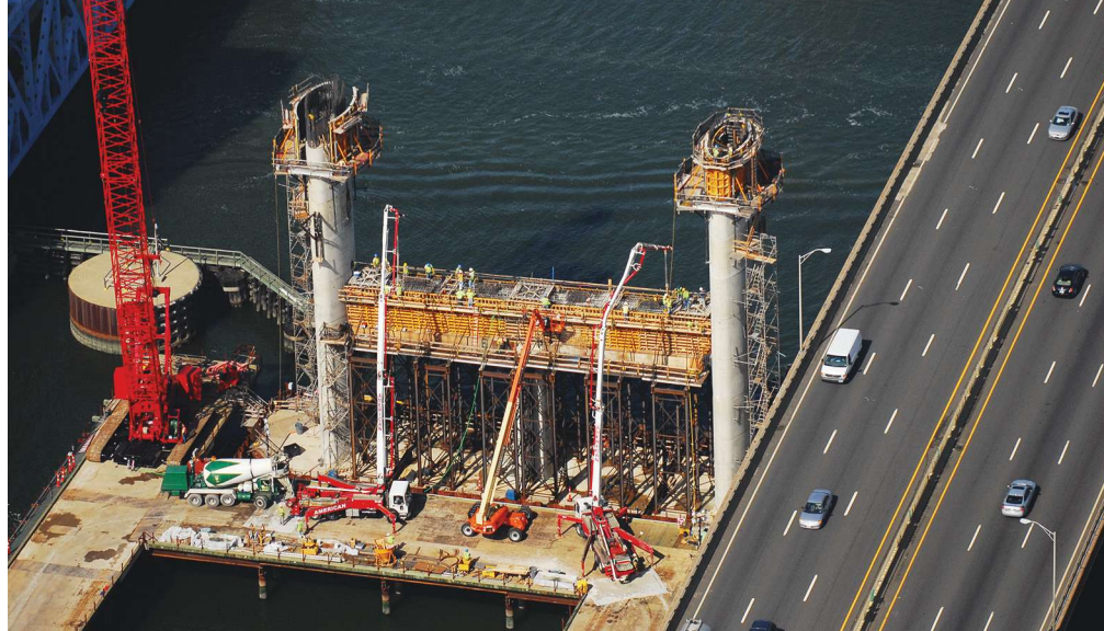
The 4649-ft-long I-95 Q-bridge, carries 10 lanes of traffic and features a 1000-ft-long main span. Photo: Walsh Group.
