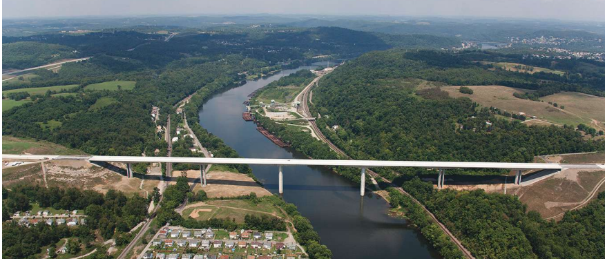
The Mon River Bridge 51H near Brownsville, Pa., features a contractor alternate design created by FIGG Engineering Group consisting of dual-cell concrete box girders. Photo: Walsh Group.
