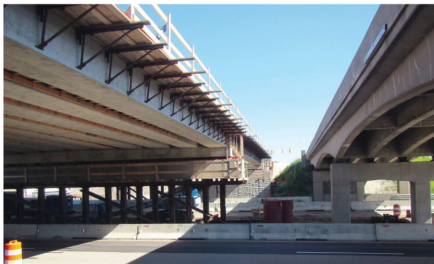
New superstructure on temporary supports (left) with existing bridge (right). Photo: Parsons.
