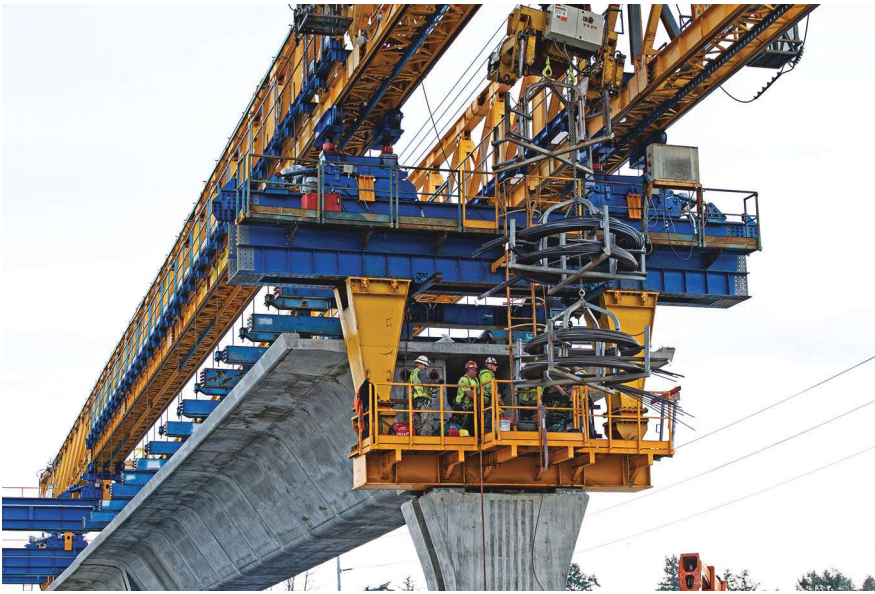
Crews prepare to launch the gantry to the next span. Photo: Roger Marble Photography.
