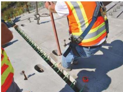
The 6-in.-wide precast concrete deck panel joints, shear pockets, and leveling coil bolts. Photo: George Bornstedt.
