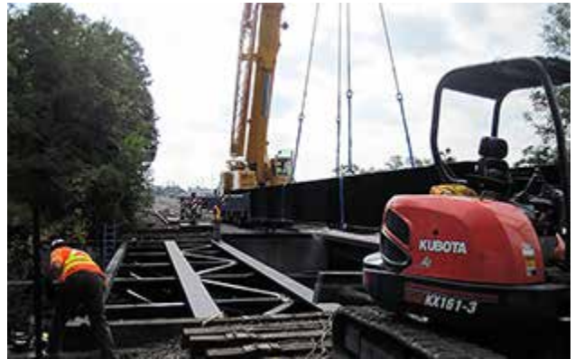
Top side view of phase construction at MBTA mile post 219.74.
